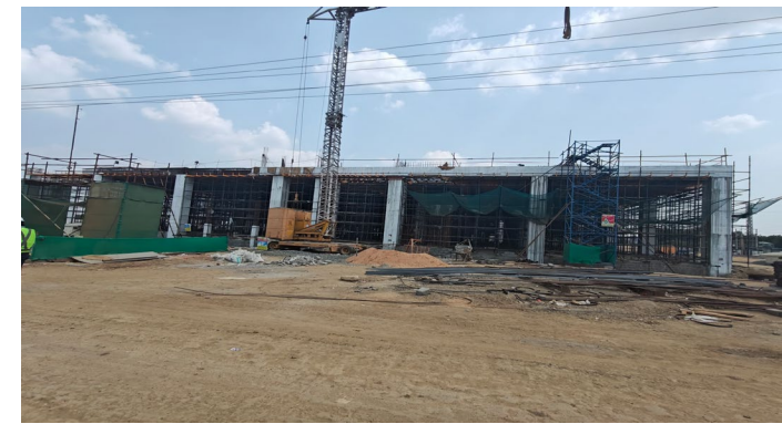
Foundation and structural work underway
